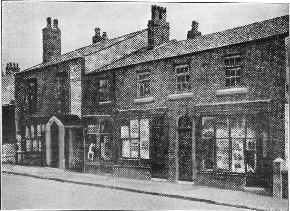
No. 100. —Church Street in the '70's. Site of Empress Buildings.
