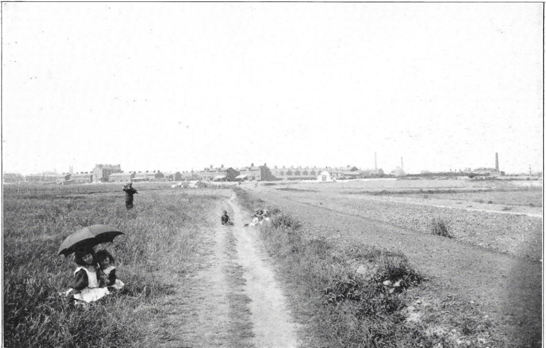
No. 160.—Central Drive.
