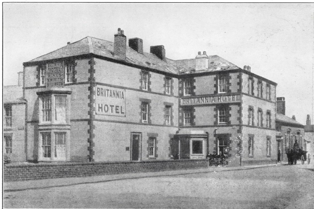
No. 140.—Britannia Hotel, South Shore.
