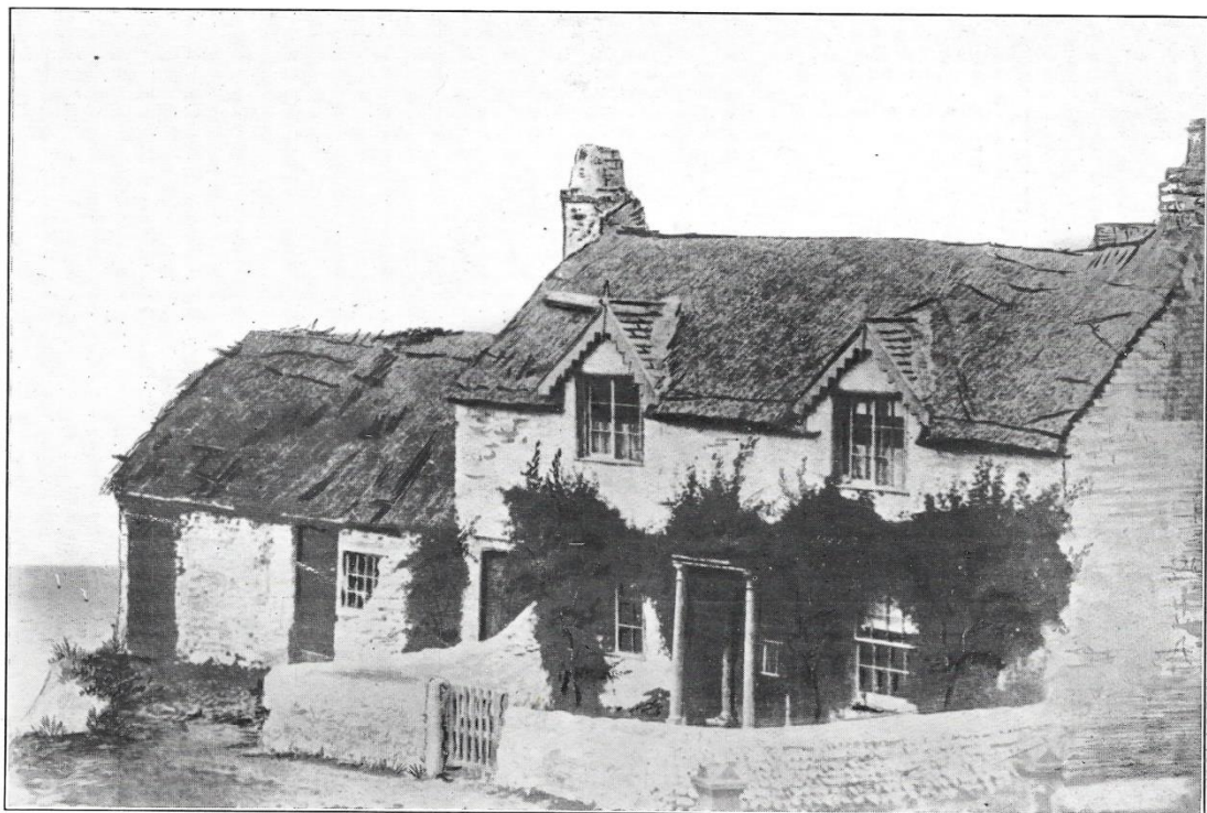
No. 67. —Cottage and Stable, west end of Cocker Street, and where the Middle Walk is now situate. Built probably end of 18th century, and pulled down about 1860.
