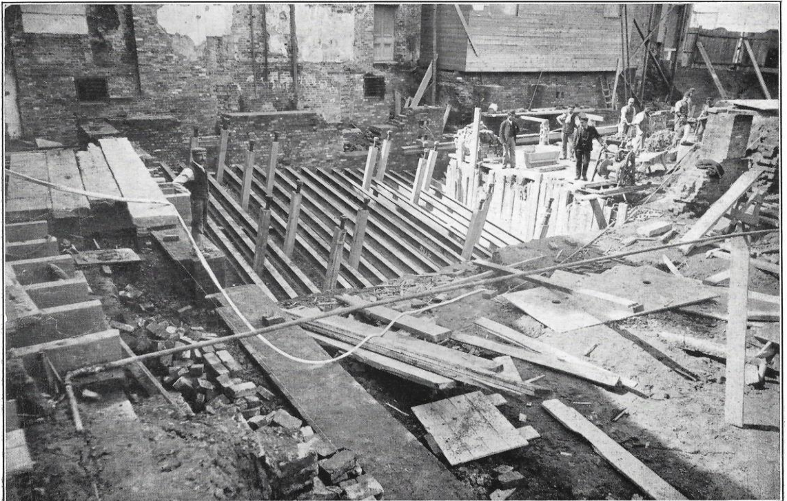
No. 176.—Foundation of the Tower.
