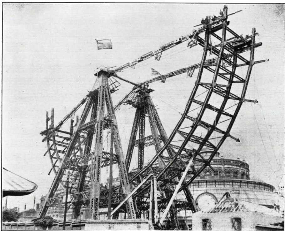
No. 208.—Big Wheel in Course of Erection.
