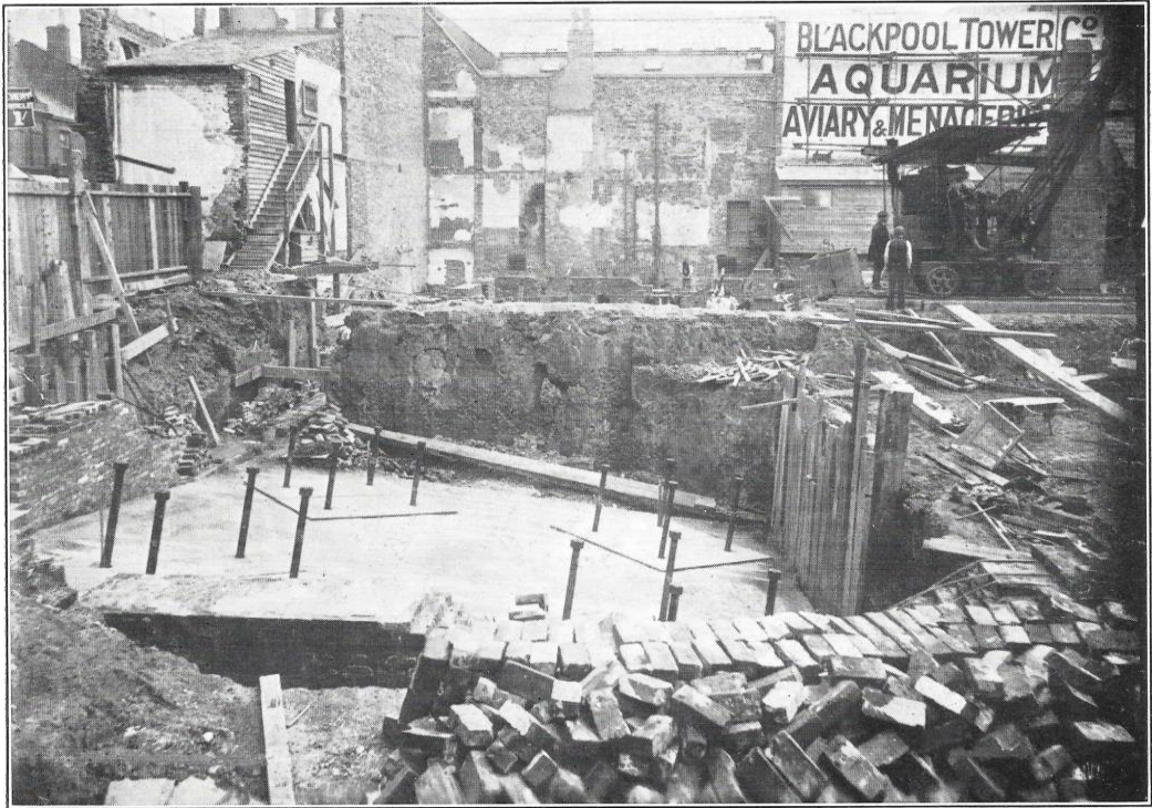
No. 175.—Foundation of the Tower.
