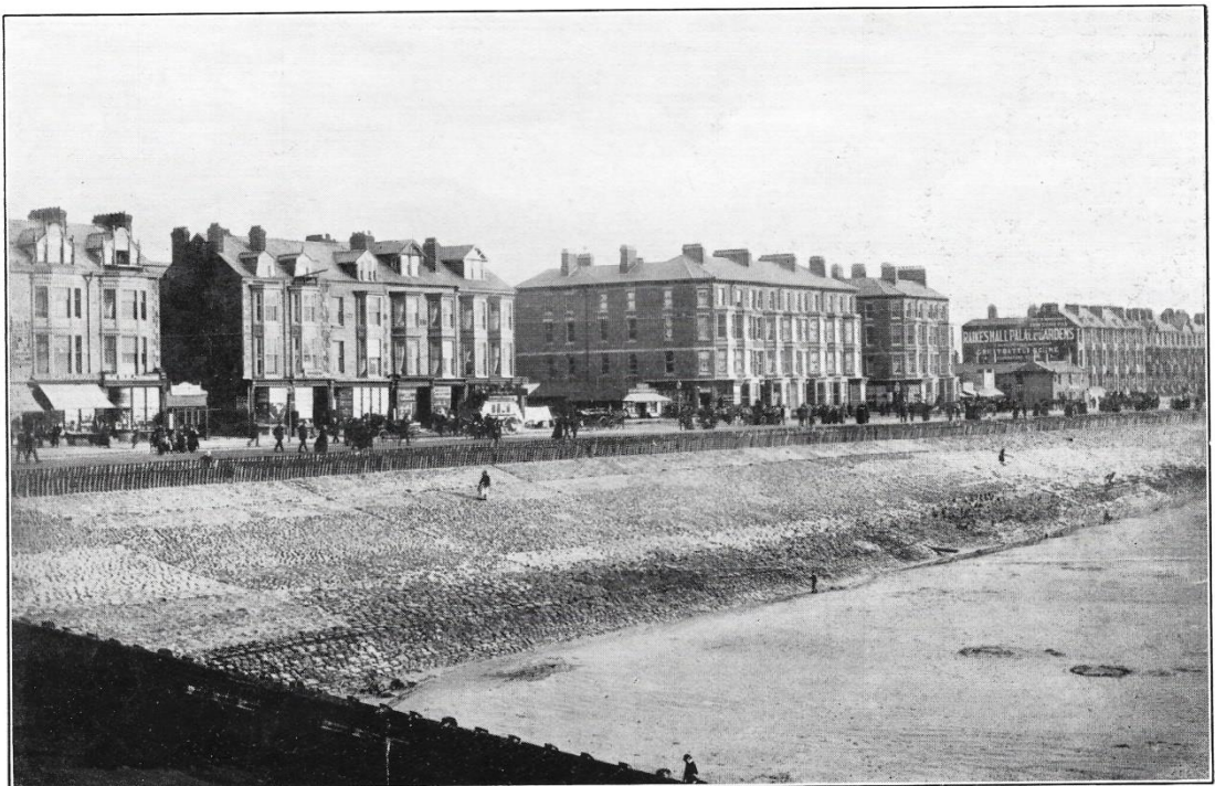
No. 204.—Looking South from Central Pier, 1890.
