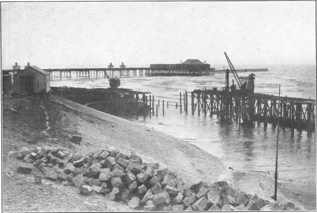
No. 241.—Driving the last piles of new Promenade, opened by H.R.H. Princess Louise, May 2nd, 1912.
